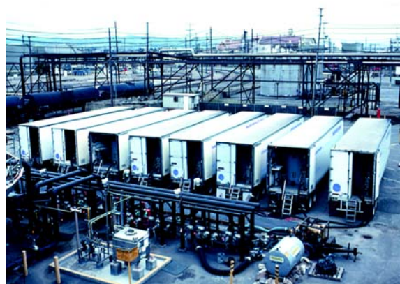
Figure 1: MobileFlow trailers used during 10-day plant repair work
