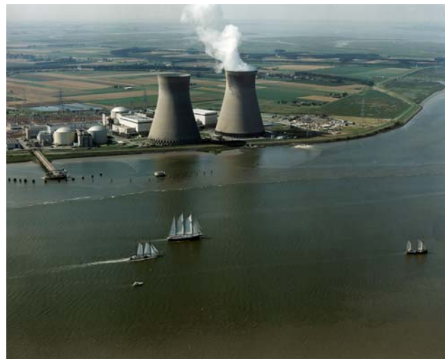
Nuclear Power Station, Belgium
