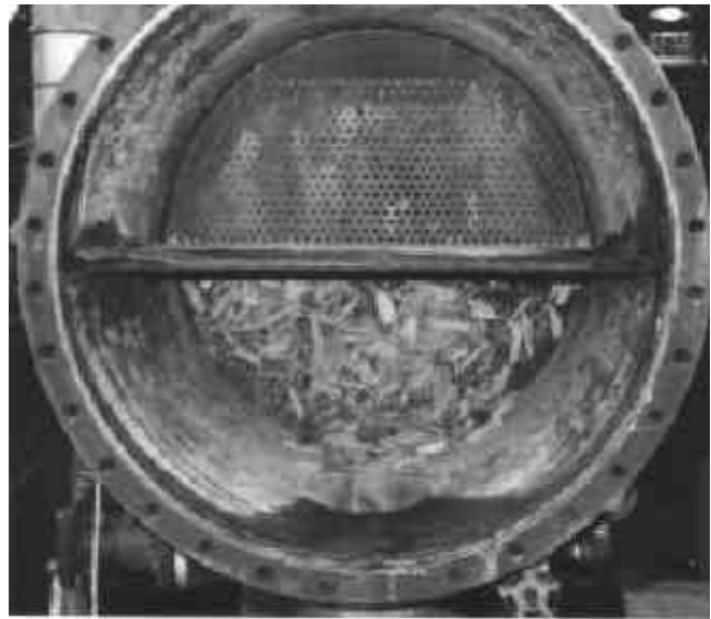
Figure 1: Exchanger Opening from Shutdown
