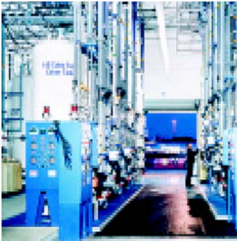
Figure 3: Interior of Facility
