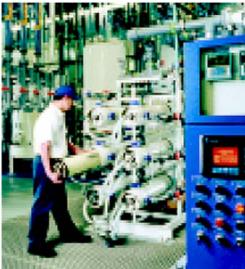
Figure 6: Interior of Facility
