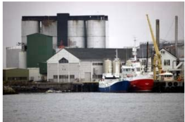
Fish Processing and Fish Oil Production Plant
